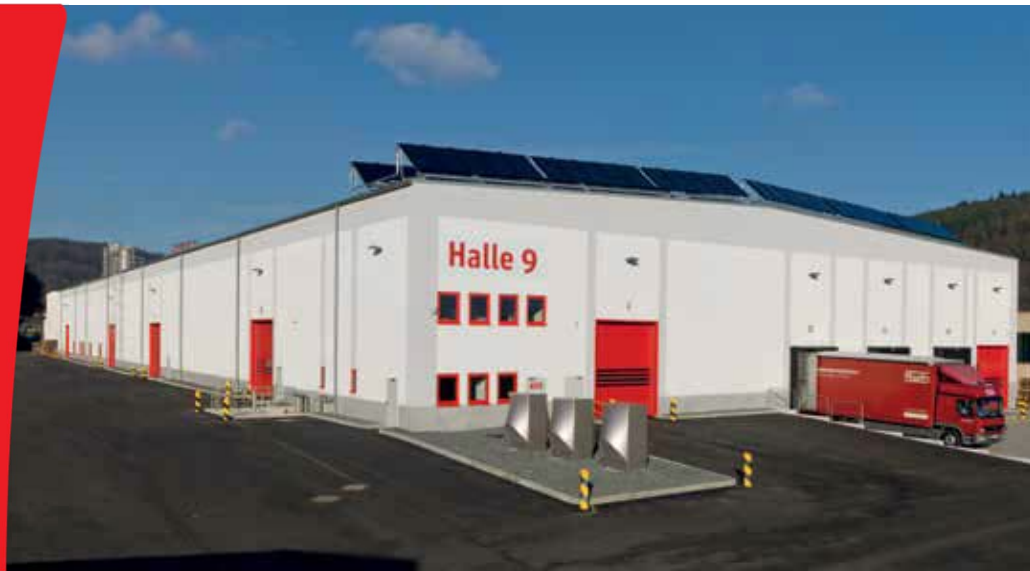
Abbildung 3 - Logistikhalle, Roth-Werke, Buchenau
